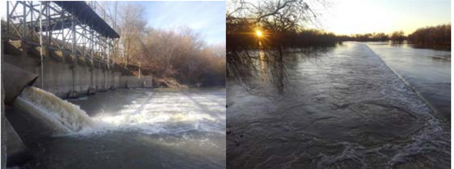
Figure 4: Examples of habitat in each of CalTrout Central Valley's fish conservation programs. Fish Food (left) pumps managed floodplain water through levees back to rivers where fish can benefit from their high concentration of aquatic invertebrates. Nigiri (right) activates floodplains in the flood bypass system and allows fish to enter. The line down the middle of the Nigiri image is the Freemont Weir being overtopped by floodwater from the Sacramento River (right of the line) and inundating the Yolo Bypass (left of the line), creating 90,000 acres of fish-accessible floodplain habitat. (CalTrout photos.)
